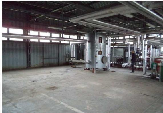
**VS92** is classic secondary exchange station supplying heating 90/70 PN 6 and hot water with central domestic hot water preparation in the heat exchange station (55°C) via 4-pipe pre-insulated pipeline into residential buildings.
