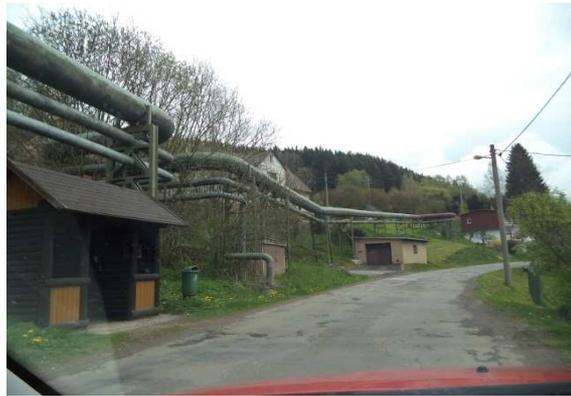
The steam line Radvanice terminates at two exchange stations. Heat is being transformed into hot water there, and subsequently distributed. The exchange stations are following:
