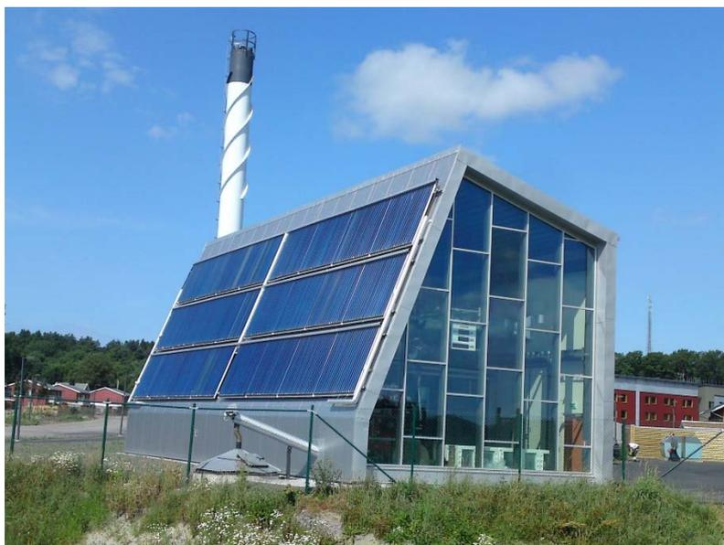
**EKSTA** has recently built a new DH system for the new residential area **Vallda Heberg** (2013). This system comprises a 250 kW wood pellet boiler, a number of buffer storage tanks and 700 m<sup>2</sup> of roof-integrated solar collectors and was realised during the course of SDH Plus (using Ritter XL collectors on the heating plant).
