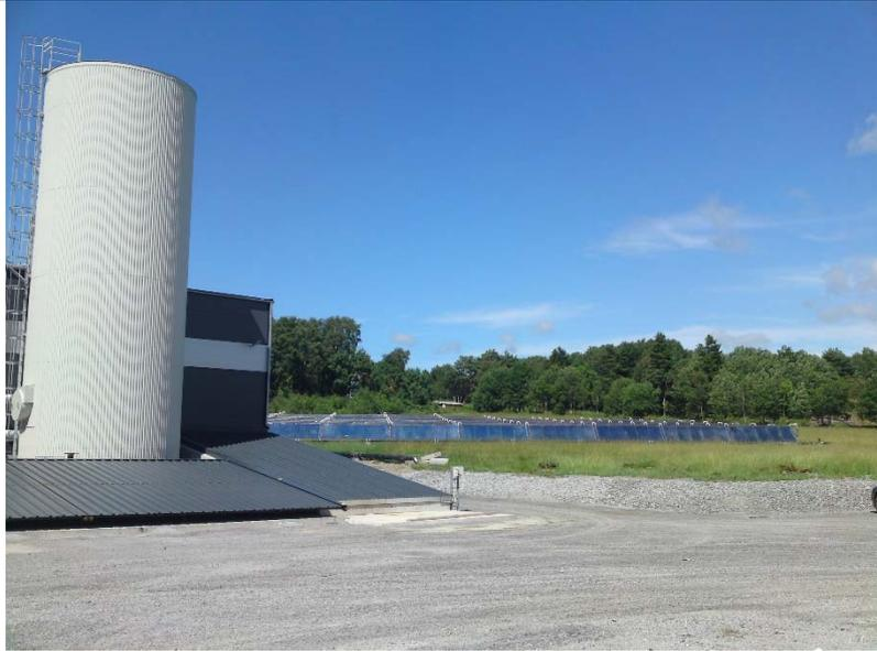
**Orust municipality** has recently built a new DH system in the village **Ellös** (2010). This system comprises a 4 MW wood chips boiler, a 200 m<sup>3</sup> buffer storage tank and 1 000 m<sup>2</sup> of (ARCON) solar collectors on ground and was realised during the course of SDH Take-Off. A national study tour to Ellös solar heating plant was organised within the SDH project in June 2015.
